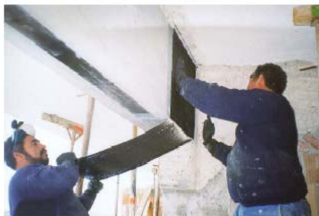
Fig. 9.5 Shear and Flexural Strengthening of a beam.
